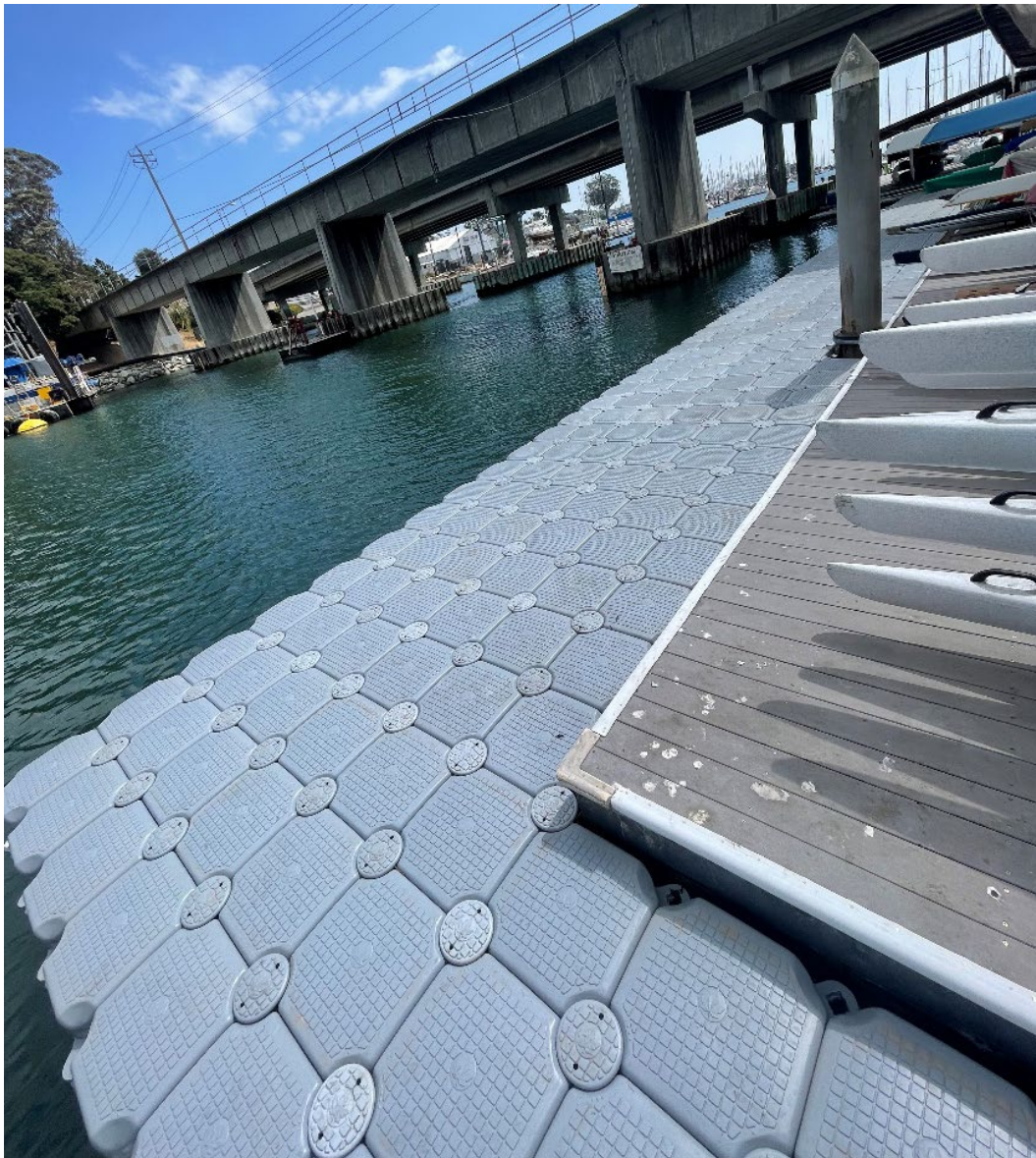
New jetfloat installed at FF-Dock.
