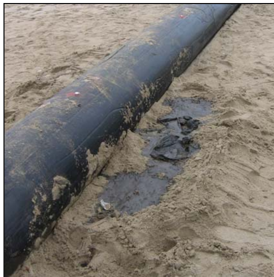
Figure 14. On the morning of October 13 th a small amount of silt and clay leaked from the dredge pipe onto Twin lakes Beach. The deposit is approximate 3 feet long and 1 foot wide and less than 0.5 cm thick.
