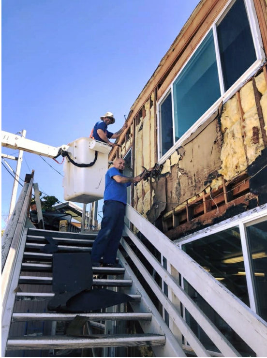
Pictured on the left: Supervising Harbor Maintenance Worker Nick Gullo and Harbor Maintenance Worker Jose Vera replacing damaged siding at 333 Lake Avenue. Not pictured, Harbor Maintenance worker Randy Marty.
